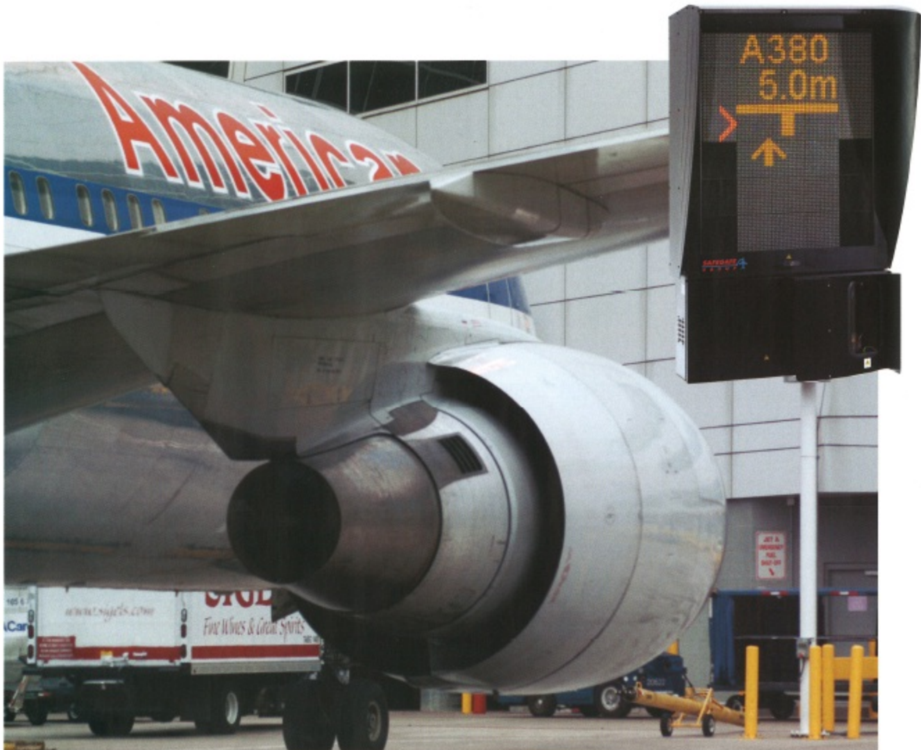
Safegate docking guidance system
